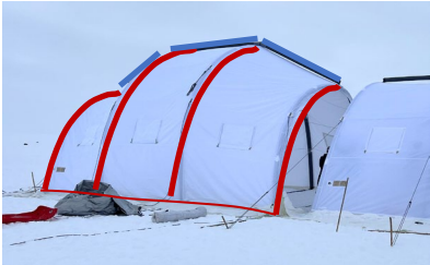
Pressure Circuits: The purlin beams and arches are on separate pressure circuits, but each circuit is linked and inflated together
